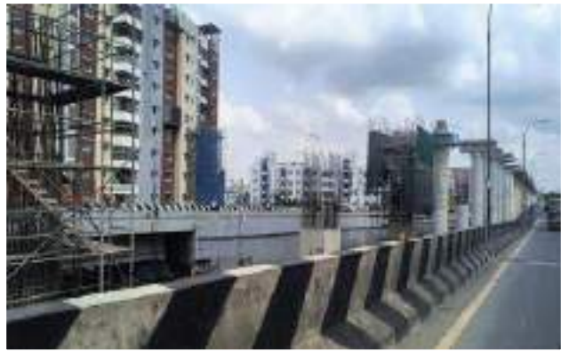
Chennai Metro Project, Tamil Nadu , India
