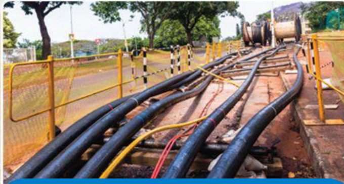
Underground Cabling Works in Rampur, Uttar Pradesh, India
