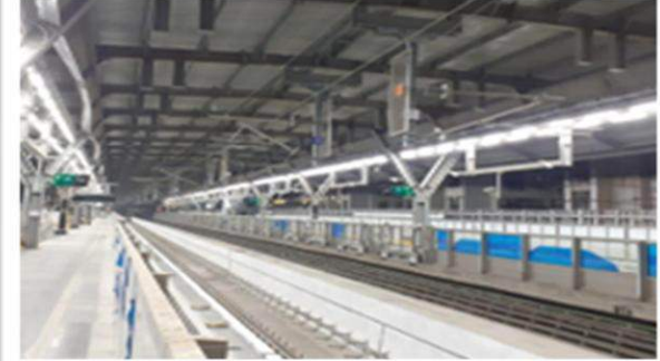
Mumbai Metro Project, Maharashtra, India
