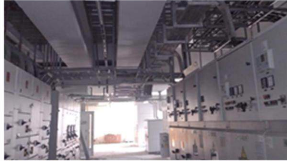
Bengaluru Metro Project, Karnataka, India
