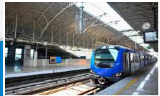
Chennai Metro Project, Tamil Nadu , India
