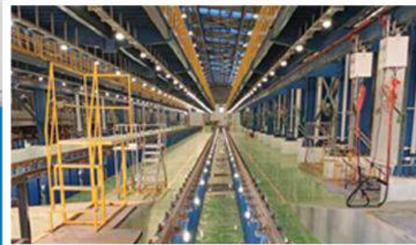
Mumbai Metro Project, Maharashtra, India
