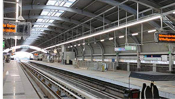
Kolkata Metro Project, West Bengal, India
