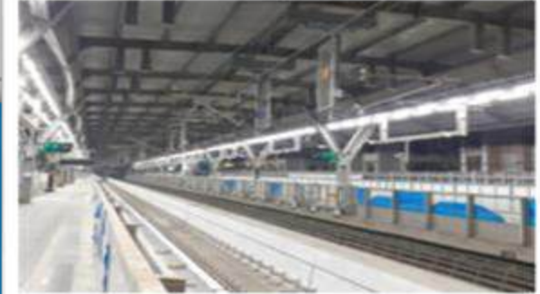
Mumbai Metro Project, Maharashtra, India
