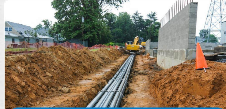
Underground Cabling Works in Maharajganj & Kushinagar, Uttar Pradesh, India
