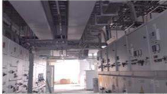
Bengaluru Metro Project, Karnataka, India
