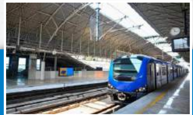
Chennai Metro Project, Tamil Nadu , India
