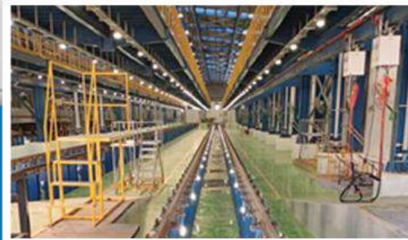
Mumbai Metro Project, Maharashtra, India
