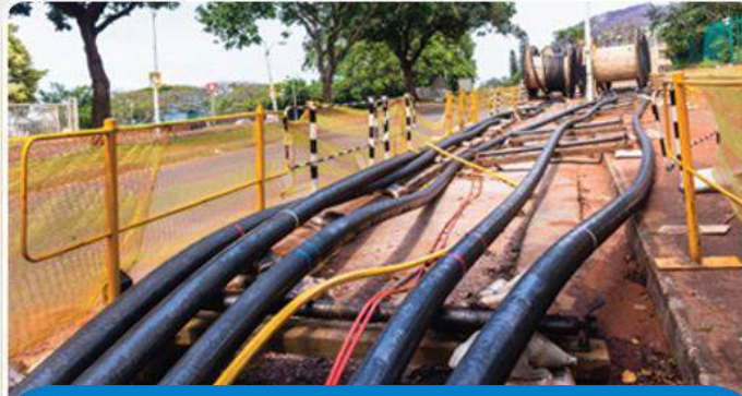
Underground Cabling Works in Rampur, Uttar Pradesh, India
