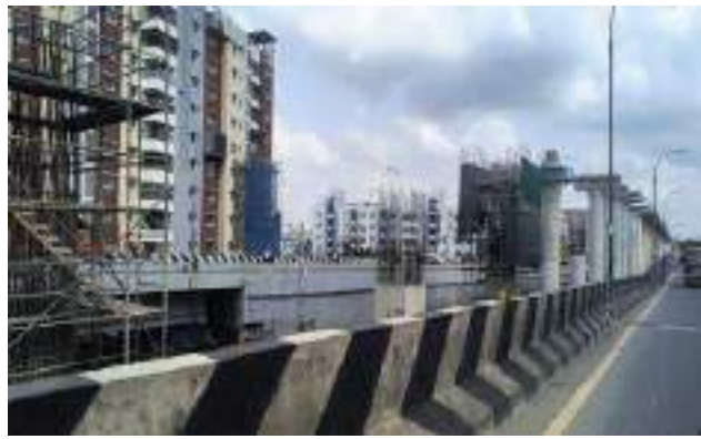
Chennai Metro Project, Tamil Nadu , India
