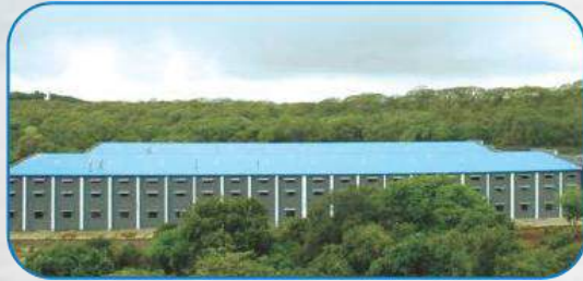
Genset Manufacturing Plant, Kalsar, Gujarat
