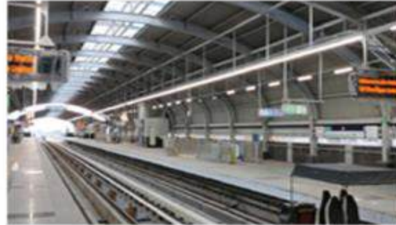
Kolkata Metro Project, West Bengal, India
